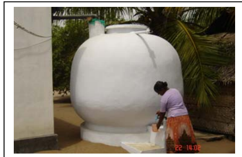
Using the rain water
